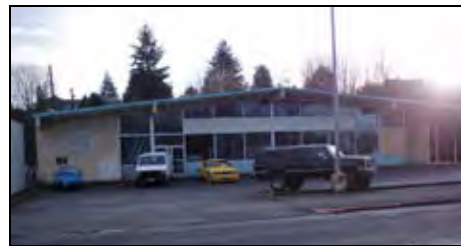
103 South Olympic Avenue
