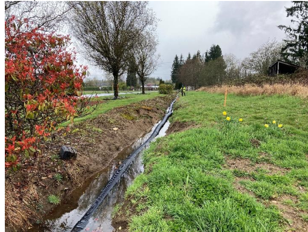
General site conditions in north ditch of the site on 04/02/24 (facing south).
