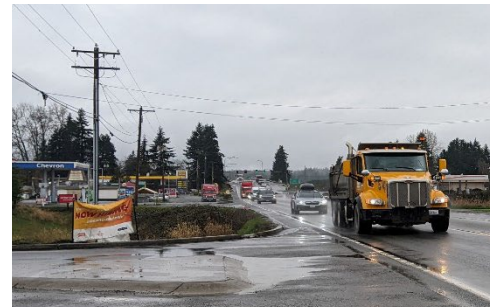
Eastbound SR 530 in the Island Crossing subarea.
