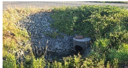
Existing culvert underneath SR 530.
