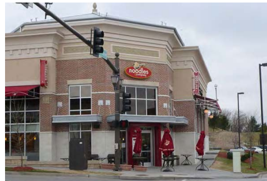
The stucco wall is located above the brick and stone wall; the brick and stone comprise at least 50% of the wall area.
