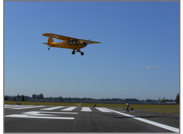
Restriping of Runway 16/34 on August 1st
